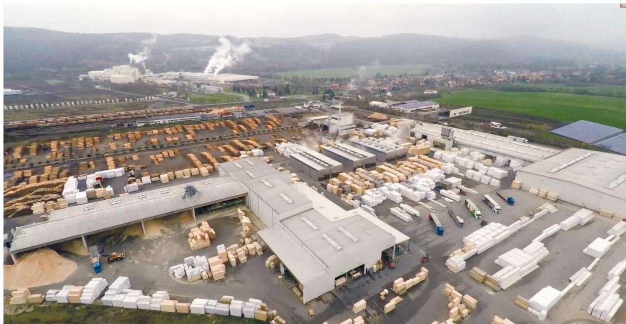
ante-holz GmbH in Rottleberode
